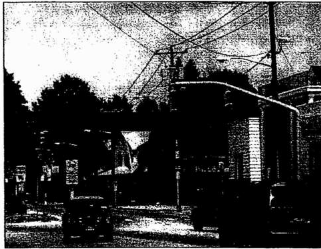
(a) Mast-Arm Mounted Signals at a Y-Intersection
